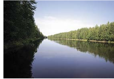
The tailrace after landscaping. Photo: Fortum Oyj photo archive (DSC 4520 w)
