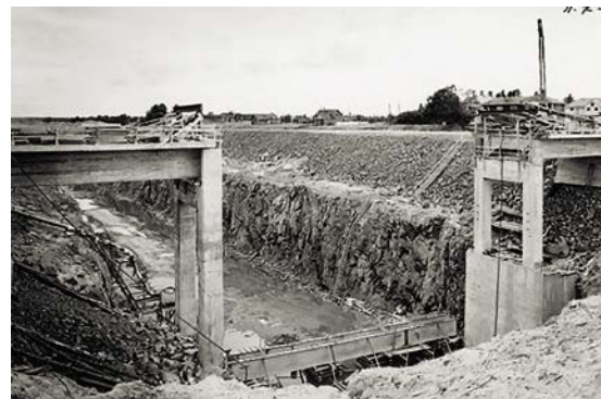
Looking down into the tailrace. Photo: Fortum Oyj photo archive (U7 263 - 11.7.1956)
