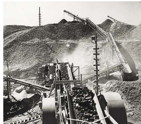
View of the scale of the excavations. Photo: Fortum Oyj photo archive (U7 256 - 10.5.1956).
