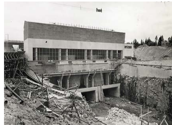
The power station and start of the tailrace. Photo: Fortum Oyj photo archive (U7 261 - 11.7.1956).
