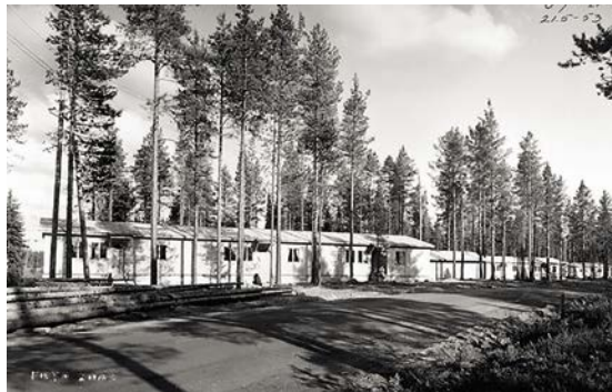
Workers' accommodation. Photo: Fortum Oyj photo archive (U7 21 - 21.5.1953)
