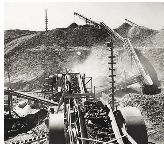
View of the scale of the excavations. Photo: Fortum Oyj photo archive (U7 256 - 10.5.1956).
