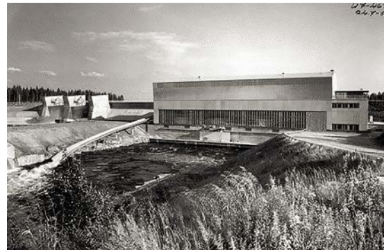
Dam on left of power station with log chute in between. Photo: Fortum Oyj photo archive (4.7.56)
