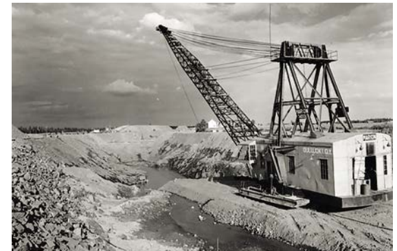
The largest crane working in Scandinavia. Photo: Fortum Oyj photo archive (U7 264 - 11.7.56)
